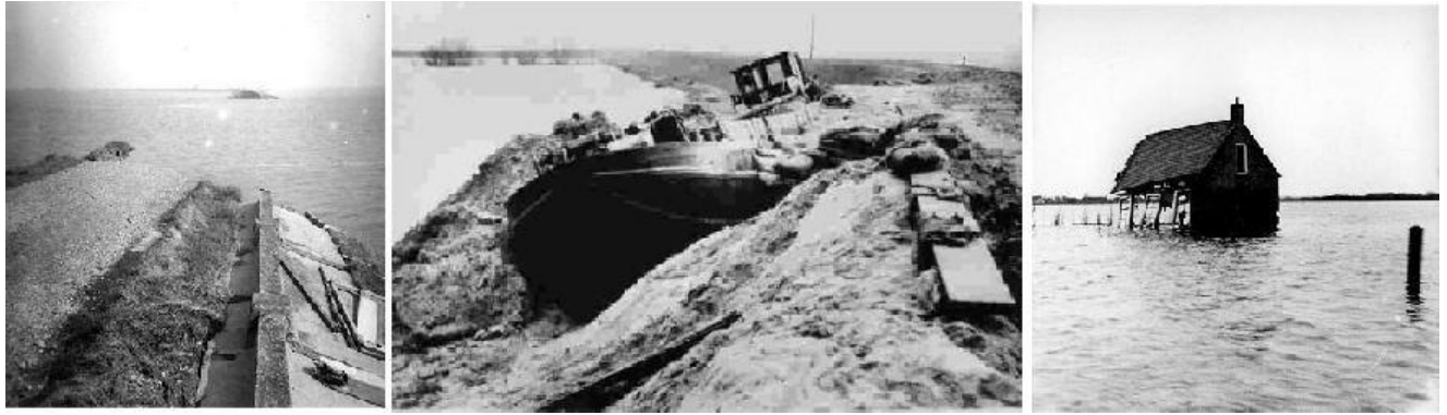
A collapsed dike after the storm (left). The river barge de Twee Gebroeders stranded in the Groenendijk dike gap (centre). A damaged building surrounded by sea water (right).
