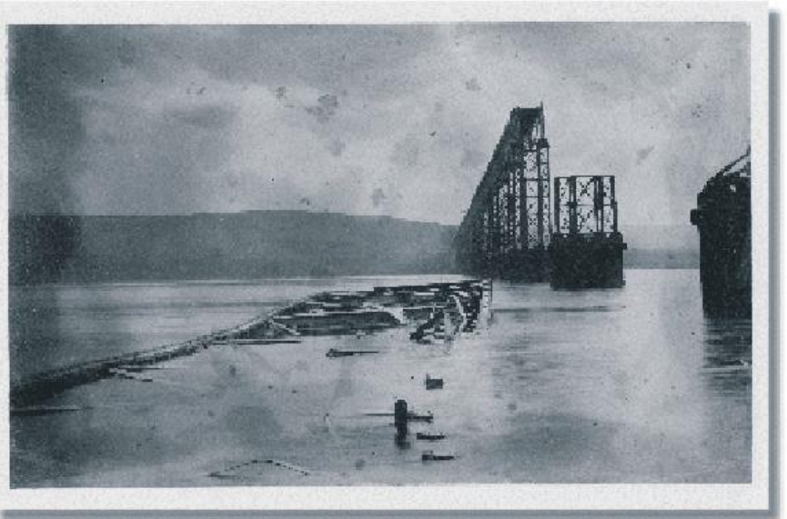
The Tay Rail Bridge disaster 28 December 1879, as documented by contemporary a contemporary newspaper (left). The old photograph to the right shows the central box-shaped section of the bridge lying on a sandbank in the river. The entire train, except for the second-class carriage and the van, was contained within this section, explaining why nobody managed to escape drowning.
