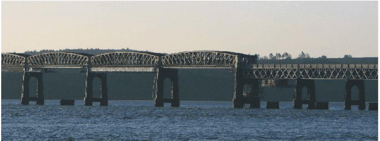
The new Tay Rail Bridge January 6th, 2008, looking SW. The old pier remains of the old bridge is seen below the modern bridge and provide a grim reminder of the 1879 disaster.
