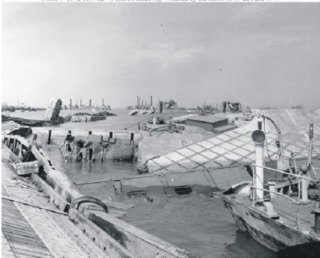
Photo # 80-G-359462 Pontoon causeway wrecked by the storm of 19-22 June 1944
