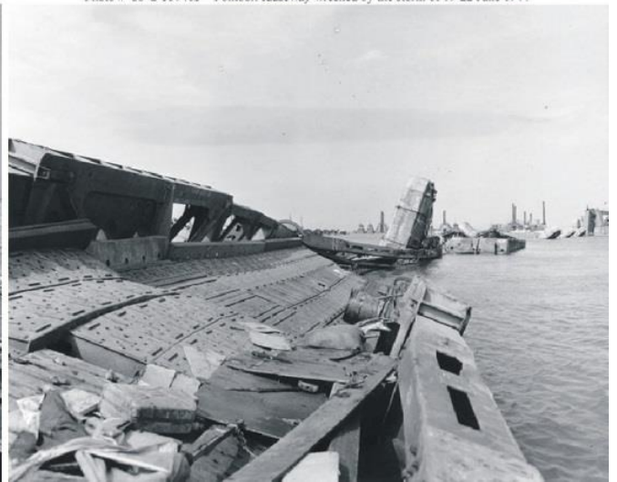
Photo # 80-G-359463 Pontoon causeway wrecked by the storm of 19-22 June 1944
